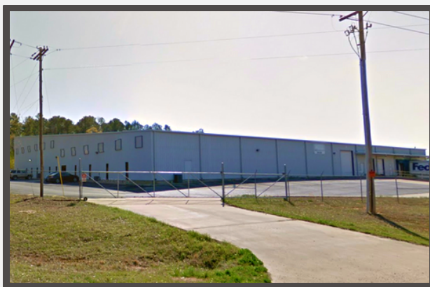
DCS Haynesville Facility (Marshall, TX)
